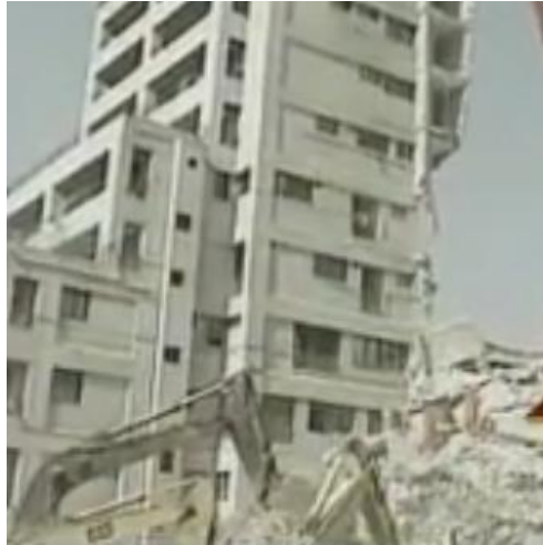
Photo 1. Collapse of Margalla Tower during Oct 8, 2005 Earthquake
