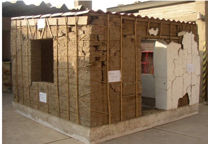
Figure 3 - External cane-rope mesh reinforcement (credits: [Torrealva y Acero et al.; 2005])
