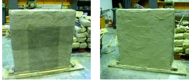
Figure 8. Strengthening of the wall with a wrapping polymeric mesh, and with plaster mortar.
