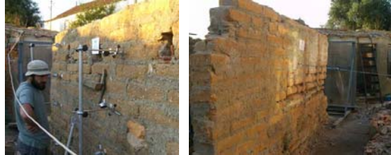
Figure 7. In situ out-of-plane testing layout: wall; horizontal displacement transducers; and horizontal loading system.
