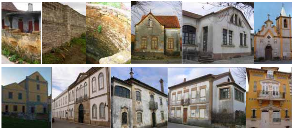
Figure 1. Examples of existing adobe constructions in Aveiro district.
