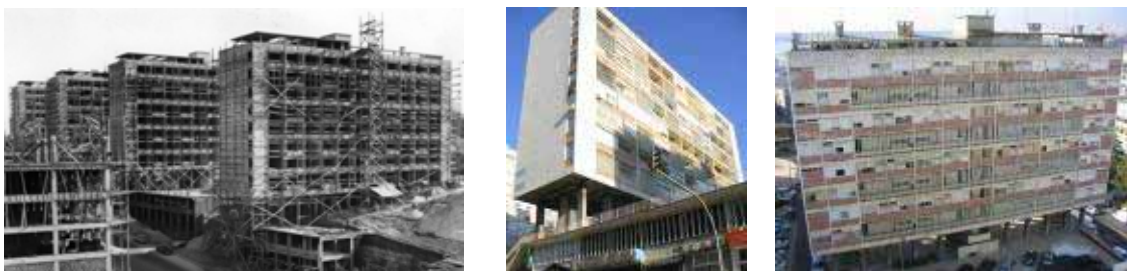
Figure 1. General views of the building block under analyses
