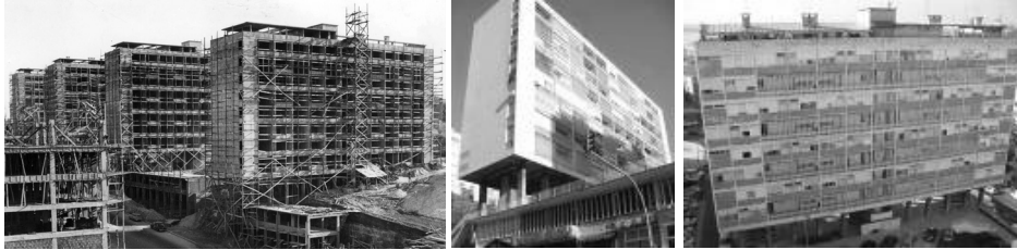
Figure 11.1. General views of the building block under analysis.
