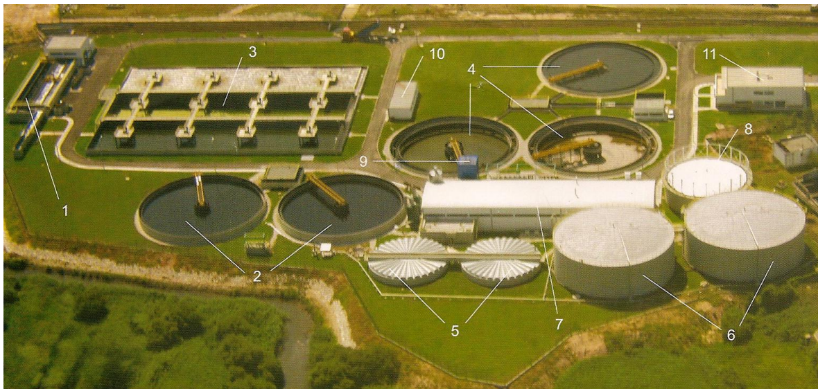
Figure 6.1. Aerial photograph of North STP (adapted from SimRia, 2011); 1– Pre-treatment building; 2– Primary sedimentation; 3– Biological treatment; 4– Secondary sedimentation 5– Sludge thickening; 6– Primary digestion; 7– Sludge treatment building; 8 – Secondary digestion and gasometer; 9– Sludge silo; 10– Transformation point and workshop; 11– Offices.
