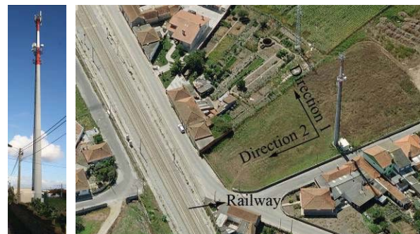
Fig. 1. a) Photography of the studied tower and b) indication of the directions for which the acceleration sensor is sensitive (the picture was obtained through Bing Maps on 7 th March 2011).
