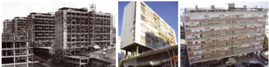
Figure 6 – General views of the building block under analysis
