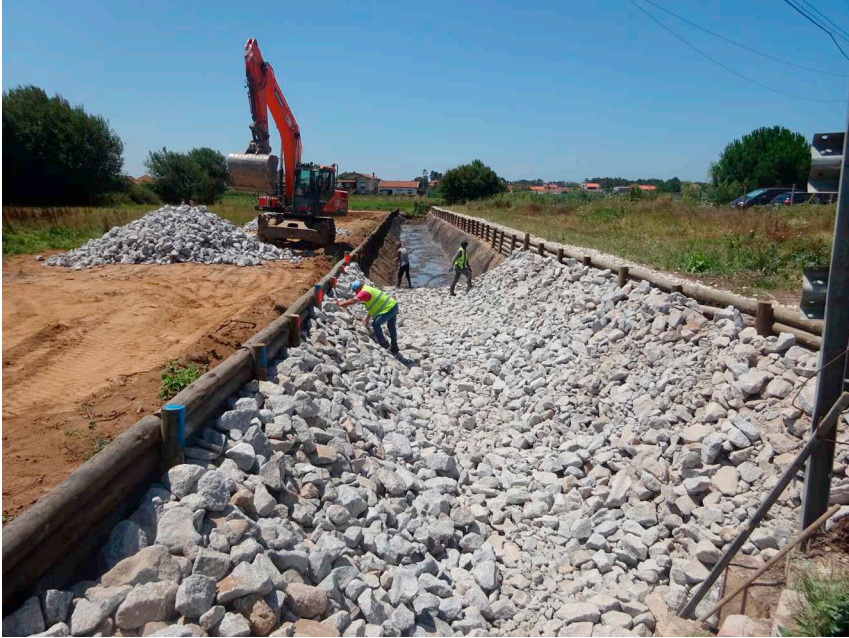
FIGURE 11.4 Paving of the ditch in the hamlet. Photograph by Fabienne Wateau 2021.
