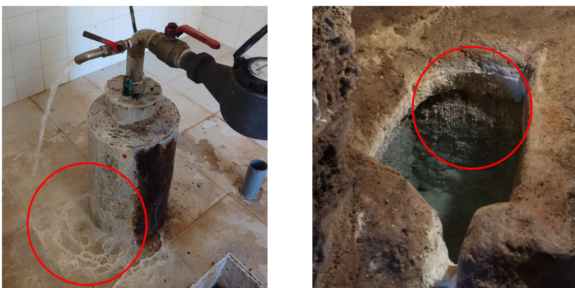
Figure 50: Calcite precipitation (highlighted with red circles) in AC5 borehole (left) and Ermida spring (right).
