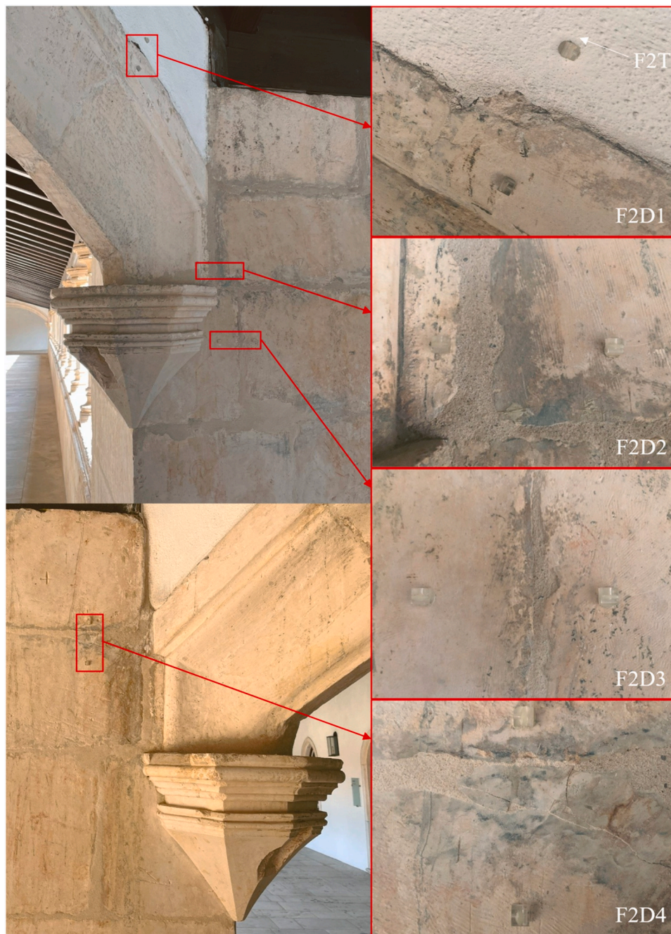
Fig. 12. Displacement sensing devices from F2 after the installation.
