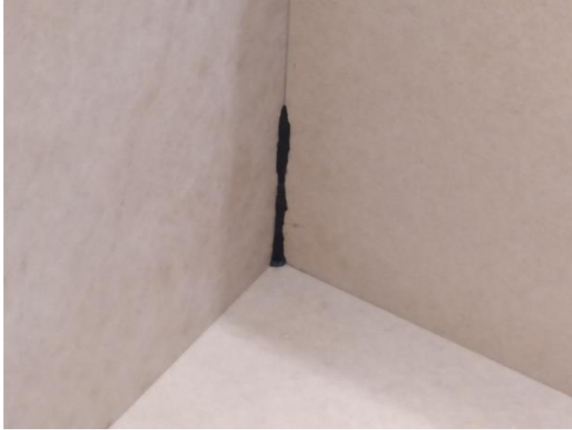
Figure 7 - Air gap covered with Alubutyl.
