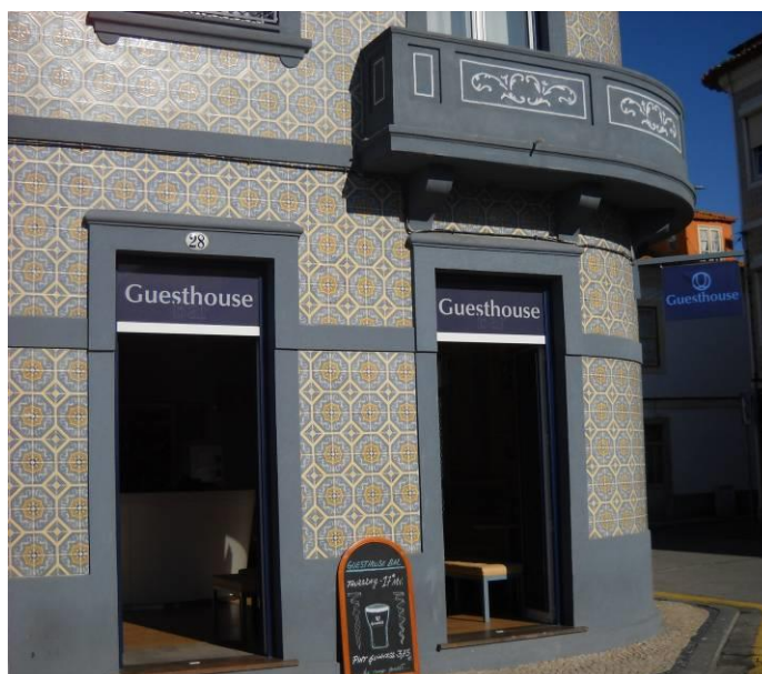
FIGURE 5 HOSTEL FAÇADE, BAR 'MORGAN & JACOB'S GUESTHOUSE'
