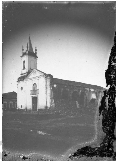
Figure 2. Partial collapse of the Nossa Senhora do Rosário dos Pretos Church, in 1974.
