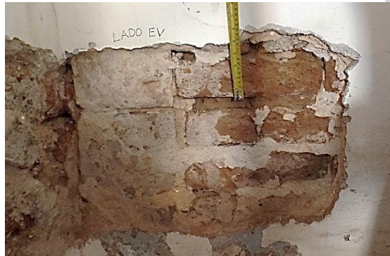
Figure 4. Detail of a clay brick masonry without mortar layer.
