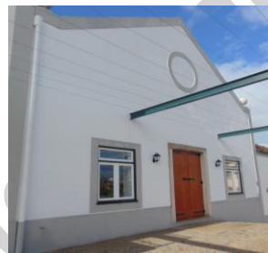
Figure 4 – Building after refurbishment
