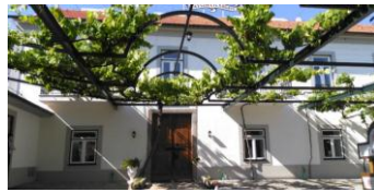
Figure 3 – Building after refurbishment
