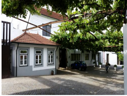
Figure 2 Building before refurbishment
