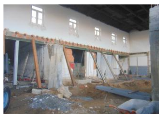
Figure 5 – Building during refurbishment
