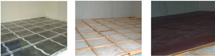
Figure 3.10: Pictures of an experimental underfloor heating system with macroencapsulated PCM, 2004 Lin et al. [23] ; left: electric layer; centre: SS-PCM layer; right: wood layer.
