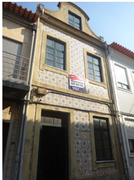
Fig. 4. Front façade of case-study building (© Alice Tavares).
