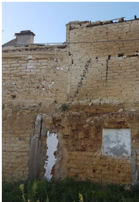
Fig. 3. Traditional wall of adobe masonry (© Alice Tavares).
