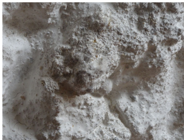
Fig. 12. Detail of salts and disaggregation in test area (image height match – 20 cm) of formed wall after seven days lime water painting (© Alice Tavares).
