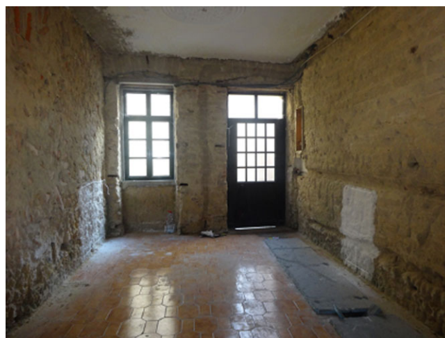
Fig. 5. Room of case-study building with lime water painting in two walls, left – formed wall; right – adobe wall (© Alice Tavares).
