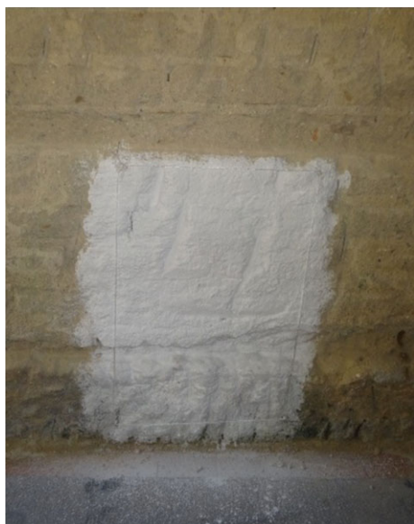
Fig. 7. General view of the beginning of the lime water application (1.0 × 1.10 m) on adobe wall (© Alice Tavares).
