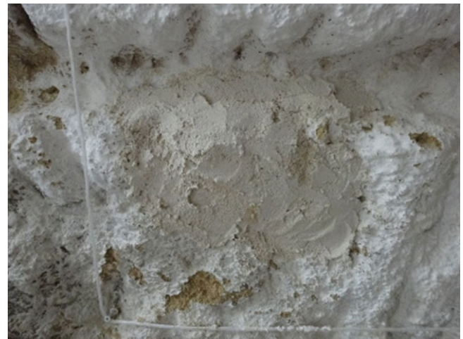
Fig. 17. Sacrificial mortar on adobe wall. Sampling sites are the yellow areas, grid size – 50 × 40 cm (© Alice Tavares).
