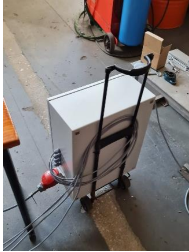
Figure 55 Wheel structure to move the electric box.
