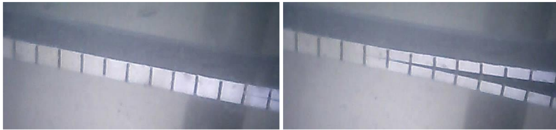
Figure 3: Image recordings with initial crack visible on the left and after crack progression on the right
