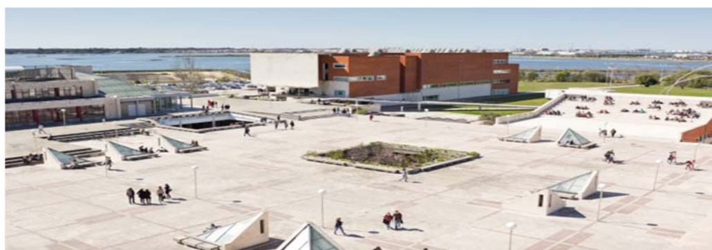
Figure 4. CTZ building roof area to be assess by the eco-design tool.
