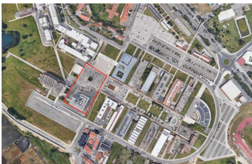
Figure 2. Central Technical Zone building localization in the University Campus.
