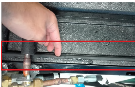
(a) Implementation of a foam strip between the EPP lid and the remaining EPP structure of the module.
