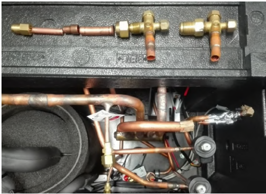
(a) CM - refrigerant circuit.
