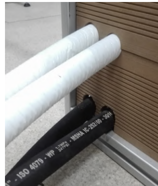
(b) Refrigerant (white) and water (black) hoses passing through the drilled holes in the WPC.
