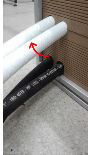
(b) Illustration of the sound leakage through the clearance around the water and refrigerant hoses.
