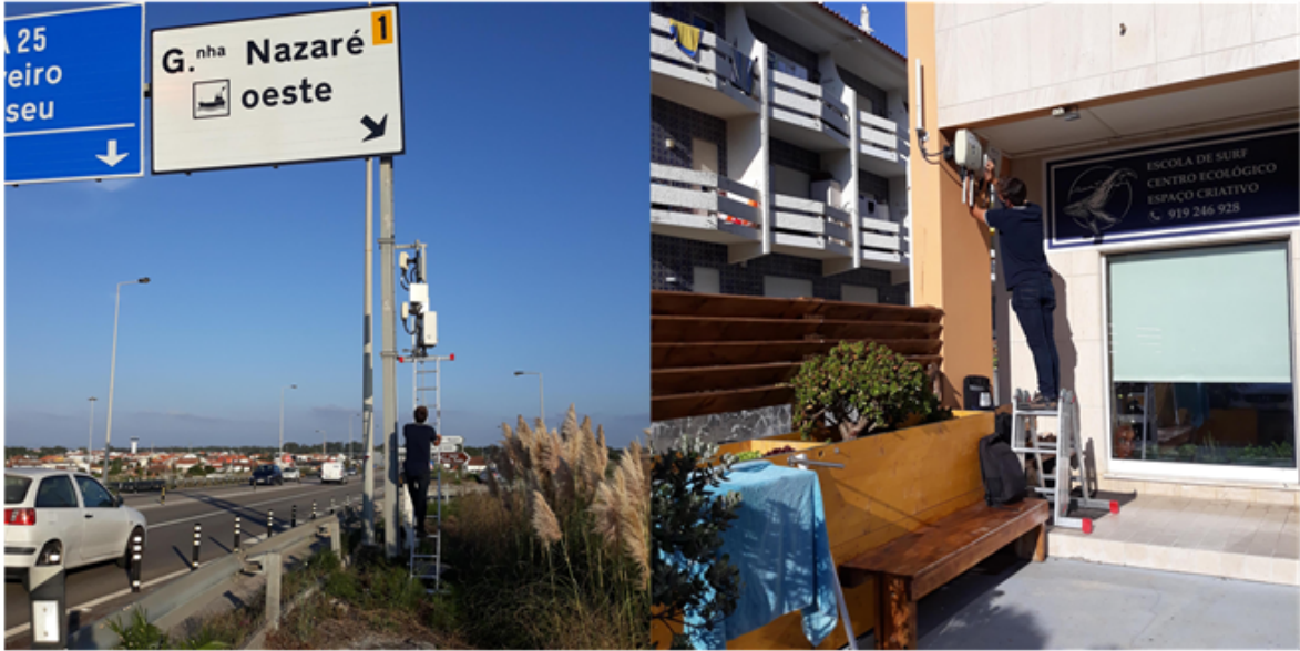
Figure 4.12: Interventions in the infrastructure
