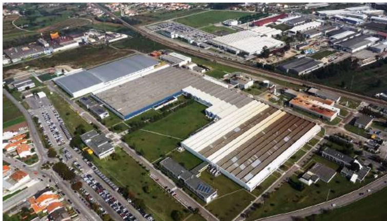
Figure 2.1: Aerial View of the Renault CACIA Plant. Sourced from: [4]
