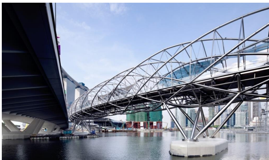
Figura 5. Ponte “Helix Bridge”, COX – Marina Bay, Singapore, 2010
