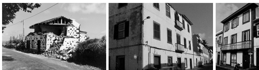
Figure 4.2: Illustration of three stone masonry buildings representative of the rural (left) and urban (centre and right) typologies of Faial Island building stock. Source: Faial database.
