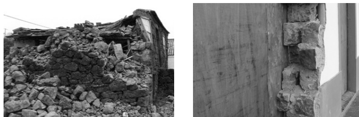
Figure 5.3: Example of the variability between rural (left) and urban (right) stone masonry typologies in Faial island.
