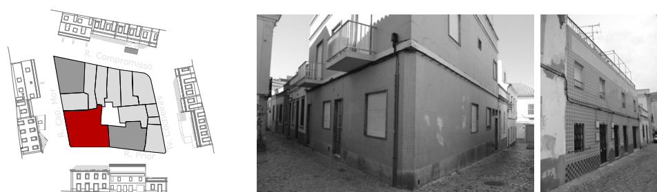
Figure 3.5: Identification of the UCH asset (in red) and of the structural units composing the aggregate: similar to the case study asset (in light grey) and distinct structural typologies (in dark grey). The pictures correspond to the structural units in dark grey.
