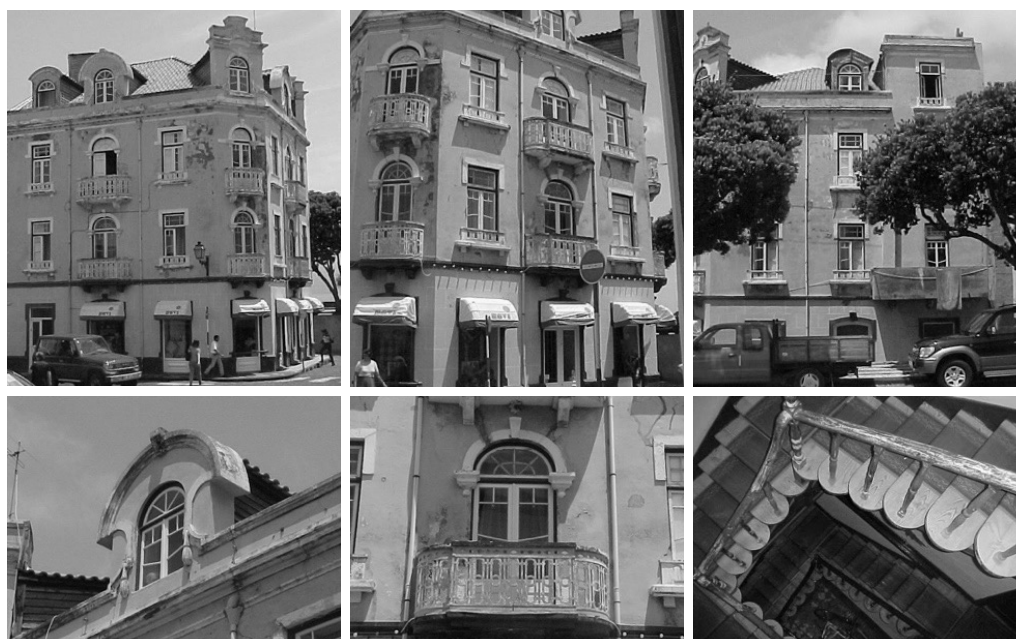
Figure 3.13: Overview of the case study building: façade walls W1, W2, and W3 (respectively from left to right in the upper row), and some architectonic details such as gable dormers, balconies and rounded openings and timber staircase (form left to right in the bottom row).
