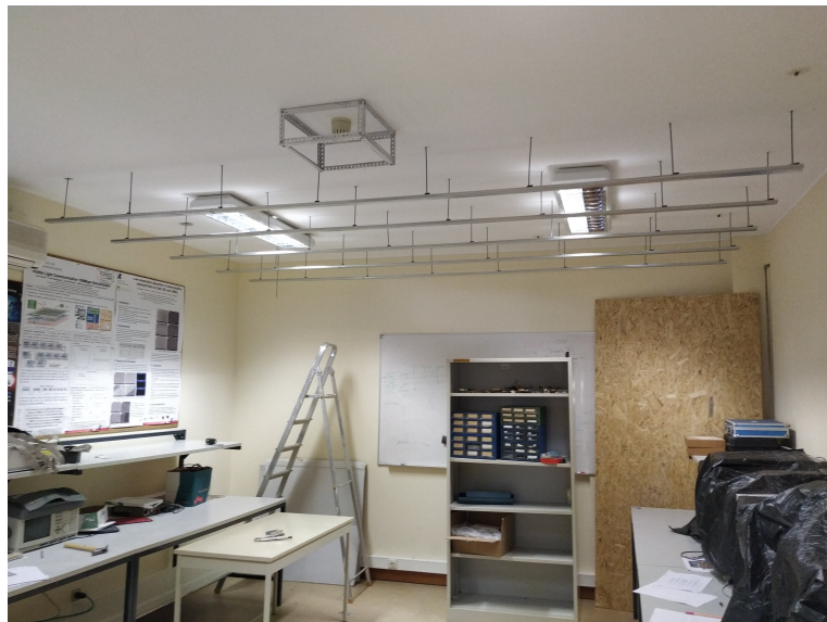
Figure 3.8: Metal frame that supports the wood panels.
