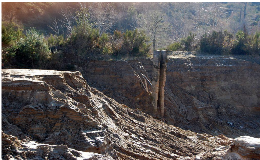
Figure 2.3 - Open impoundment with rejected material in Borralha mine. http://www.phytosudoe.eu/en/s3-borralha-montalegre-po/
