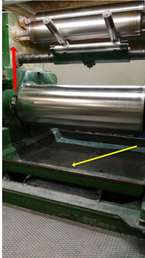
Figure 36 - Mixing cylinder and potential contamination areas
