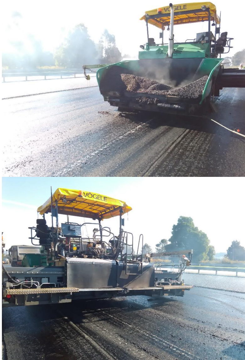
Figure 4.5 – Asphalt Paver Front/Rear
