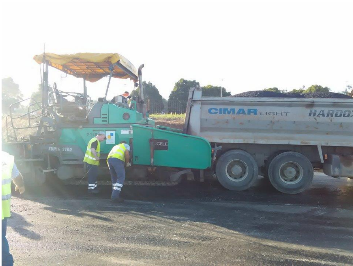
Figure 4.7 – Paving Process in Action
