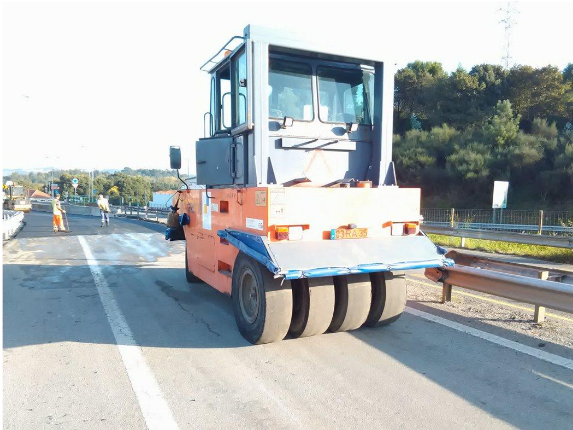
Figure 4.10 - Pneumatic Tired Roller
