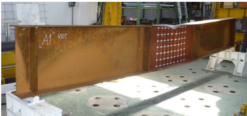
Figure 1.1: Example of local buckling of a beam after an experimental test at 450°C carried out at Czech Technical University [1.3].
