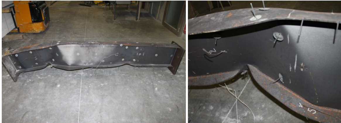
Figure 1.2: Local and global buckling on a beam-column tested at elevated temperatures carried out at University of Liège [1.3].
