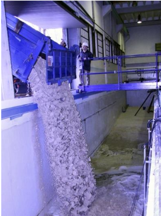
a) Sand-bed construction.
