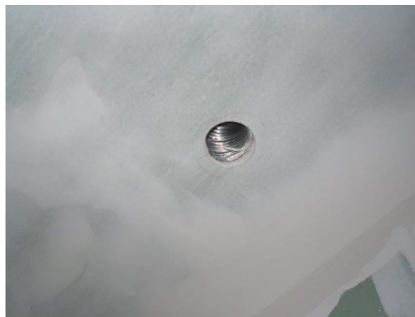
Figure 38 – Hole for the ventilation duct.
