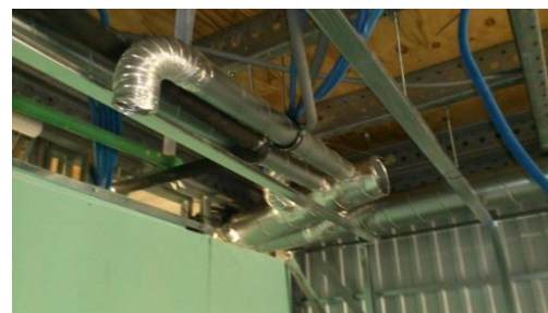
d) 2 nd floor air extraction collector
