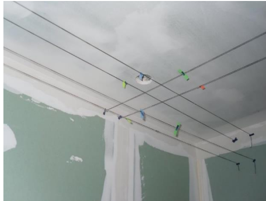
Figure 44 – Part of the grid used to mark the exact points where the anemometer registered values below the ventilation opening.
