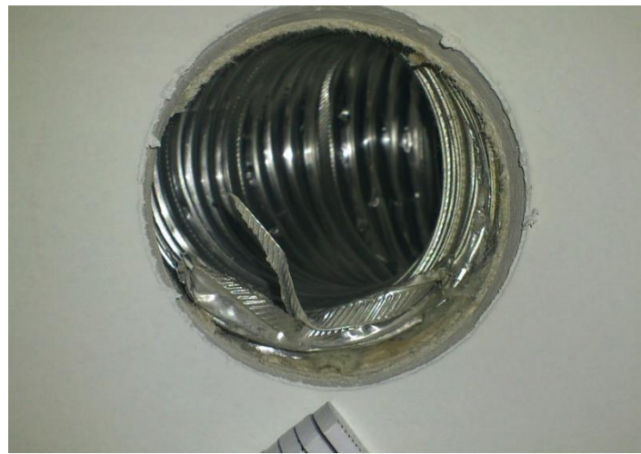
Figure 46 – Slope of the ventilation duct.
