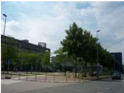
Construction of the main square – the Hafen Platz
