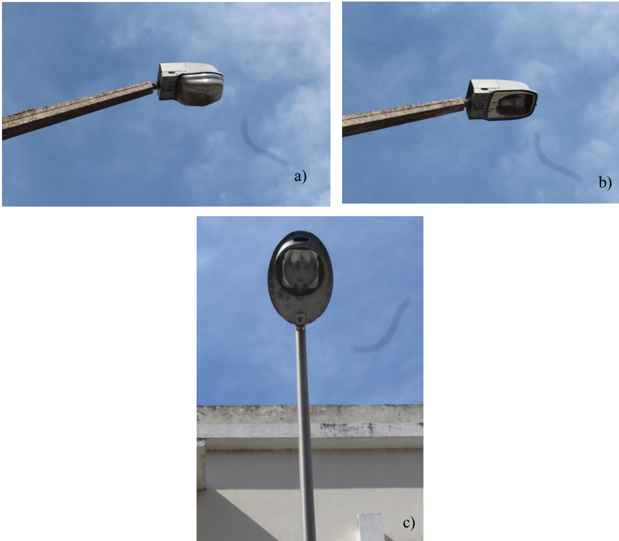
Figure 18: Luminaries of the different posts with the 250W a) with protection cover and b) without protection cover and c) the 150W luminaire.
