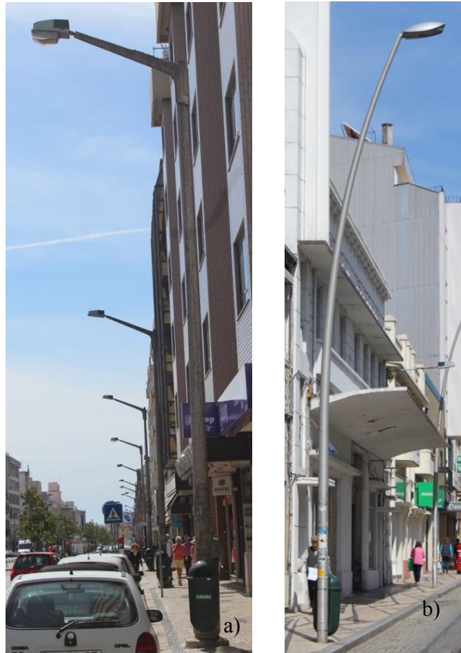
Figure 19: Posts installed in the avenue, a) 250W and b) 150W.
