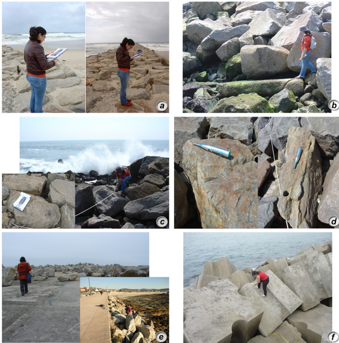
Figure 49. The overall monitoring along the maritime structures (Espinho, Vila Praia de Âncora): from the basic observation (a, b, e) to several applications of methods and tools to evaluate each sector (c, d, f).
