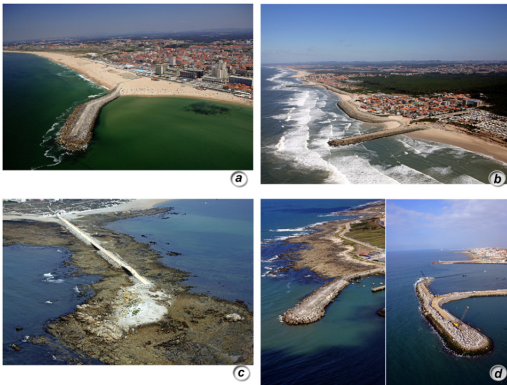
Figure 104. Examples of the coastal environments considered in this thesis: (a) sandy beach and field of groynes in Espinho (NW Portugal); (b) mixed environment (sandy beach, groynes and seawall) in Cortegaça (NW Portugal); (c) mixed environment (rocky coast, sandy beach and groyne) in Aguiño (NW Spain); (d) mixed environments in Vila Praia de Âncora and Douro River (NW Portugal). (image credits: FotoEngenho).
