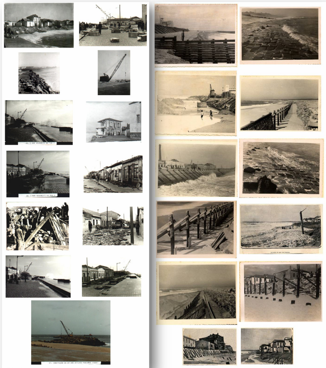
Figure 96. Compilation of images used to verify the occurrences identified on the GIS based project in Pires et al. (2007) research; some examples of the sea invasions, destruction of buildings, reinforcement of marine works; several types of coastal interventions and solutions held along the shoreline (Espinho City Council Archives, 1958-1960).
