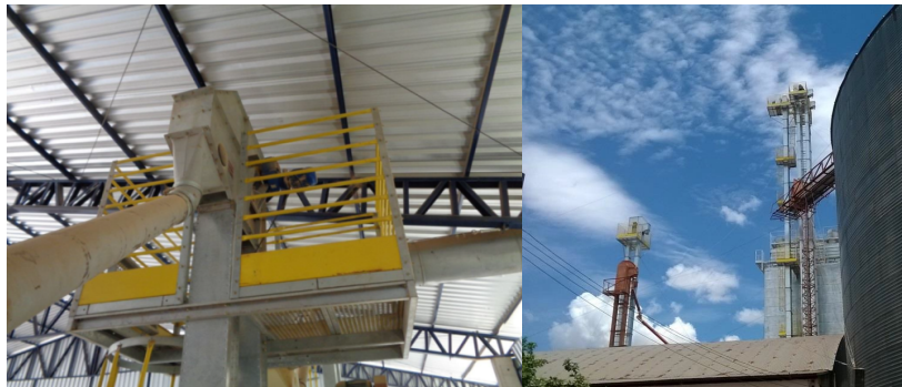
Fig.10 Installed platform in client.
