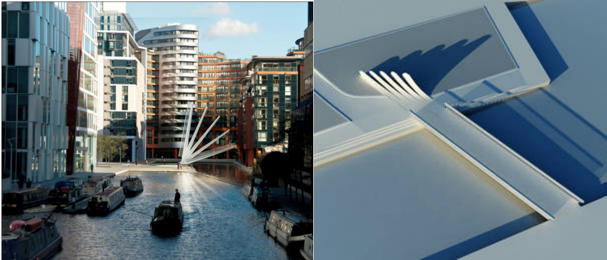
Picture 9. Merchant Square footbridge in Grand Union Canal, England (pictures from [7]).
