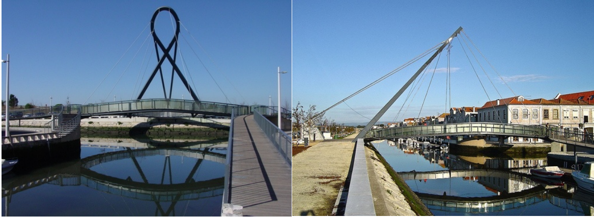
Picture 16. Circular footbridge, Aveiro, Portugal
