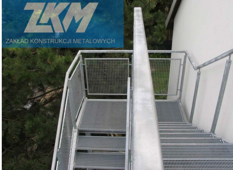
Picture 25. Steel stairs
