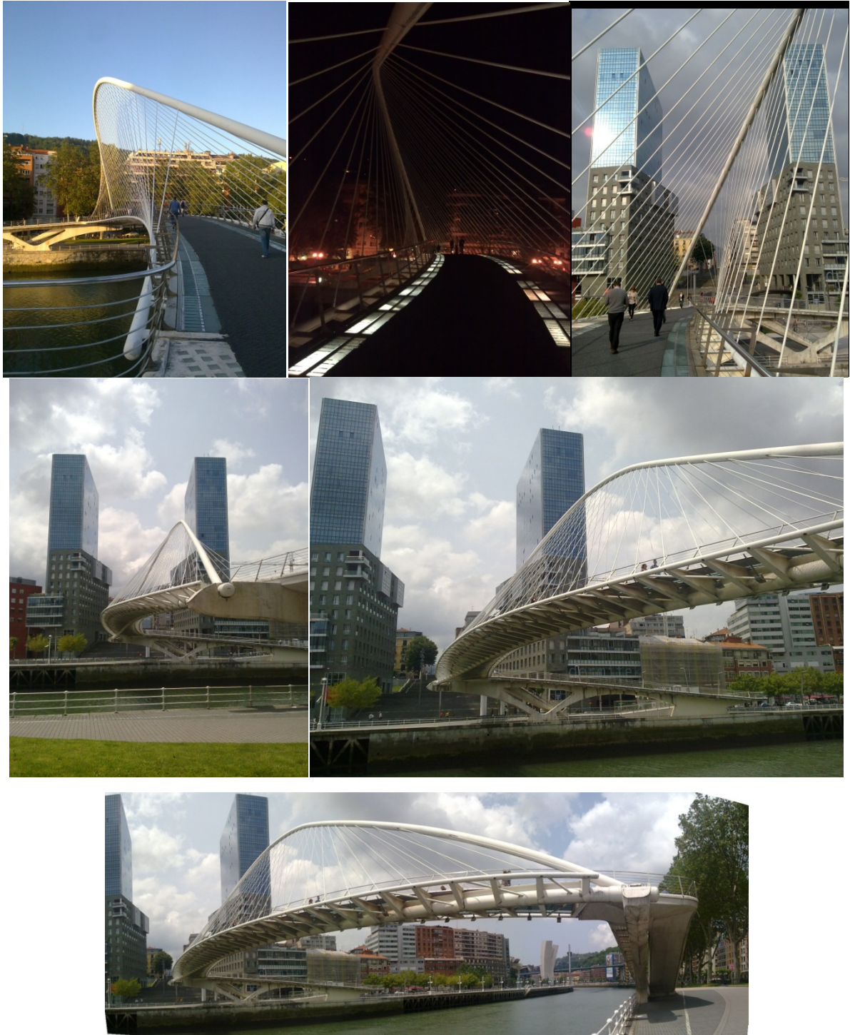
Picture 15. Calatrava footbridge in Bilbao, (pictures courtesy of Prof. Dr. Nuno Lopes)
