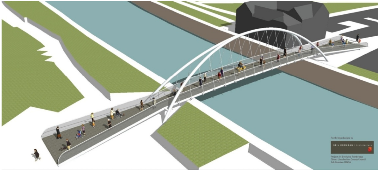
Picture 20. Arch structure footbridge
