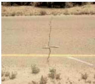
Figura 9 - Fenda transversal (Alves, 2007)
