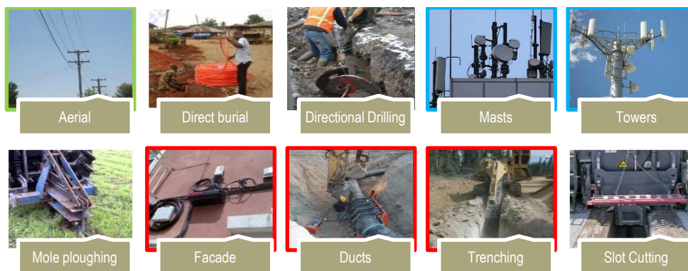
Figure 90 – Some telecommunications network's installation techniques.
