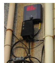
Figure 108 - Façade optical distribution point, ODP (the grey box) Source: Photo from the author.
