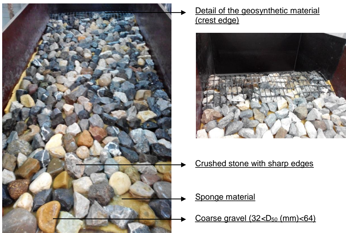
Figure 51. Foundation layer lying down at the hydraulic model channel bottom.
