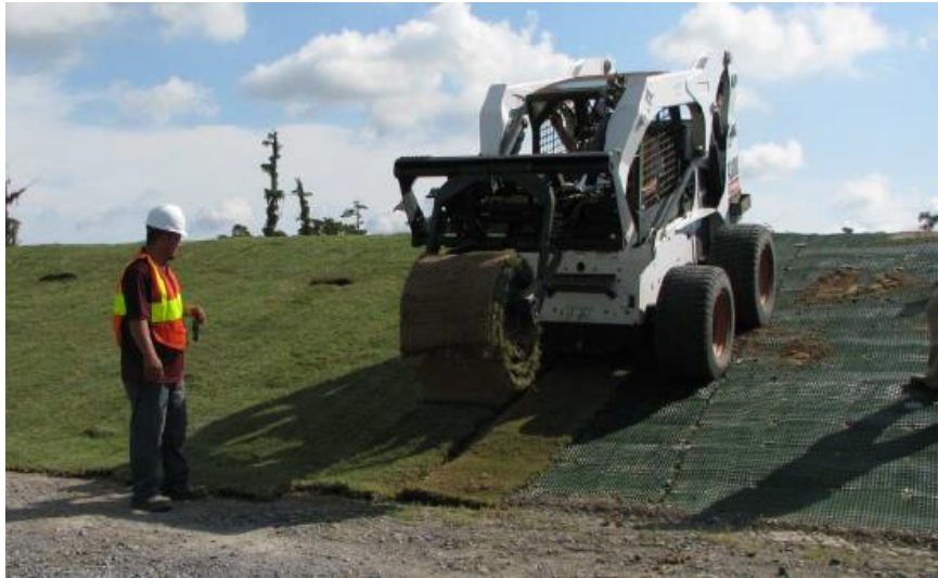
Figure 27. Installation of HPTRMs on a New Orleans dike (Flikweert et al. , 2013).
