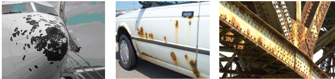
Figure 1 – Corrosion around: airplanes, cars and bridges
