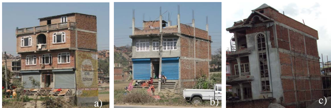
Fig. 5 Existing RC building construction practices in Nepal
