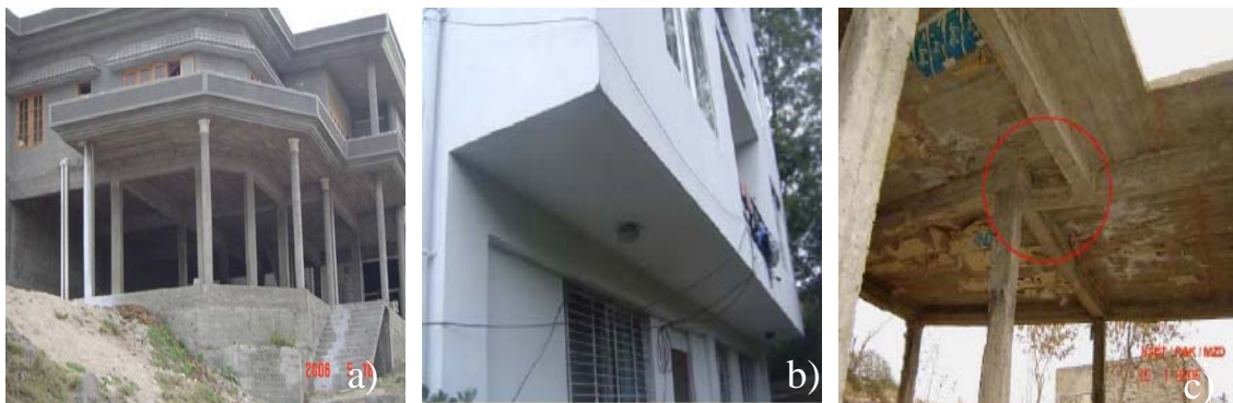
Fig. 2 a) Defective stirrups due to 90° bends joint b) Inadequate lap length c) Large spacing of lateral ties in column with 90° bend d) Column reinforcement is too short for the continuity of the column
