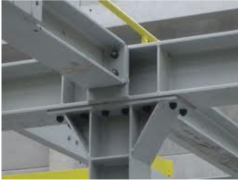
Figure 18 – Bolted connection (wiki.mech.uwa.edu.au)
