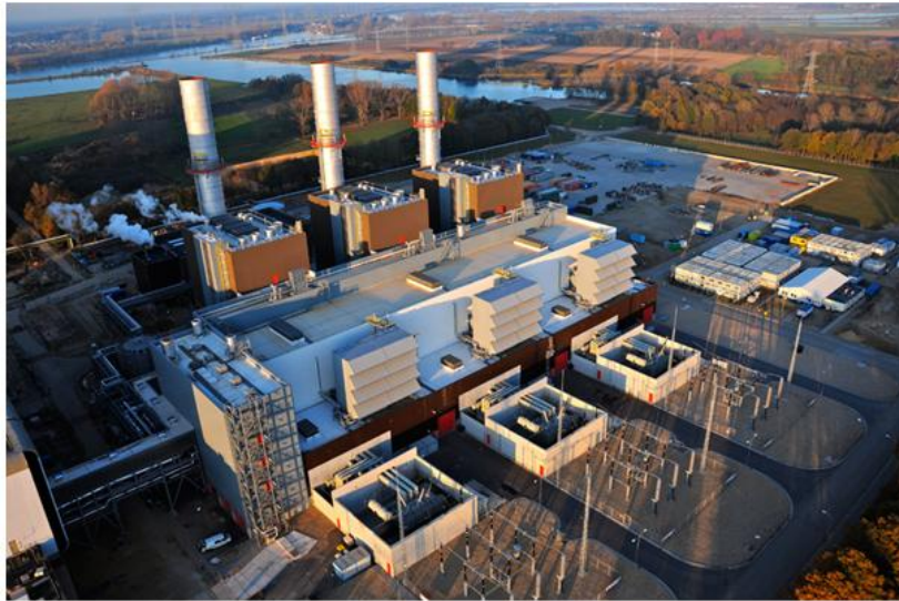
Figure 4 –Alstom Gas Power Station with three gas turbines ( www.alstom.com )
