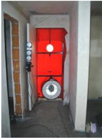
Airtightness test device. [27]
