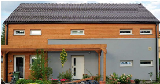
View from east side. [22]
