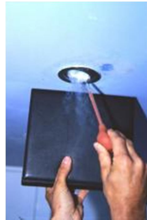
Detecting leaks after the airtightness test. [13]
