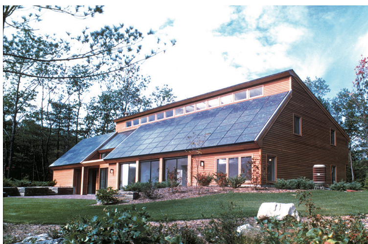
Figura 2. Net-Zero Energy Solar Home “Carlisle House” [16].
