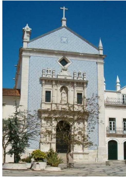
Figure 2. Main elevation of the church.
