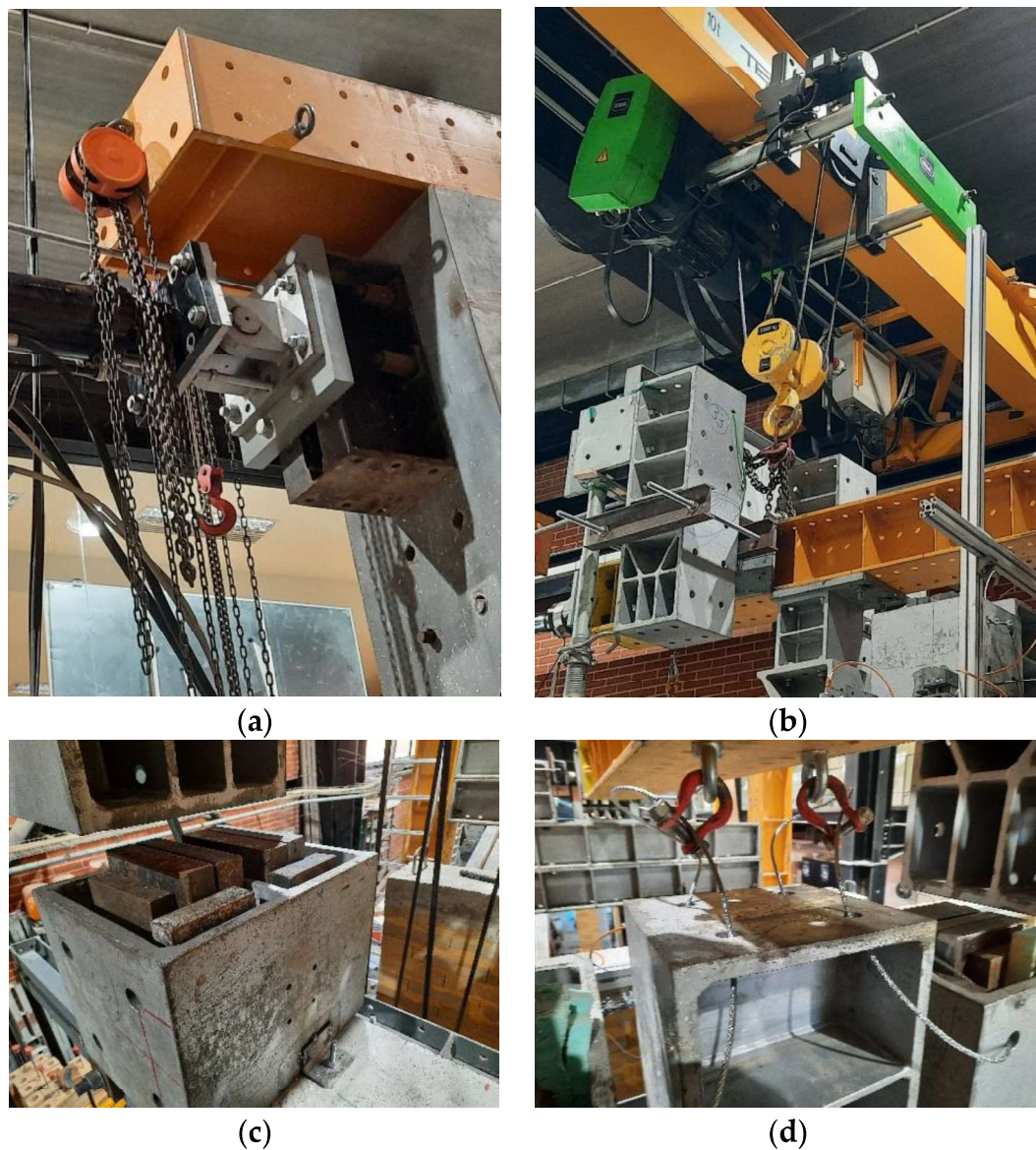
Figure 18. Details of the safety devices on the actuator (a) on the main beam (b) and on the specimen (c,d).
