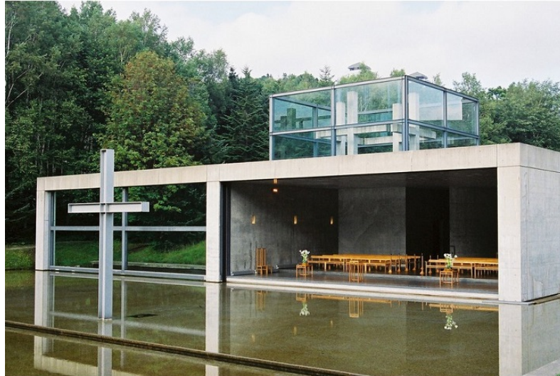
Figure 60. Church on the water by Tadao Ando 24
