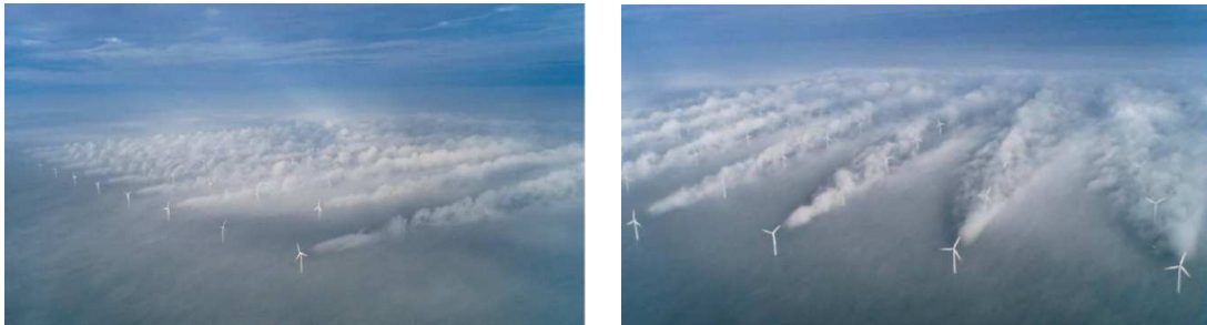
Figure 2.1.2: Wake effects behind offshore wind turbines at the HR1 wind farm (Hasager et al., 2013). In these photos it's very easy to observe how the generated wakes span to other downstream wind turbines.
